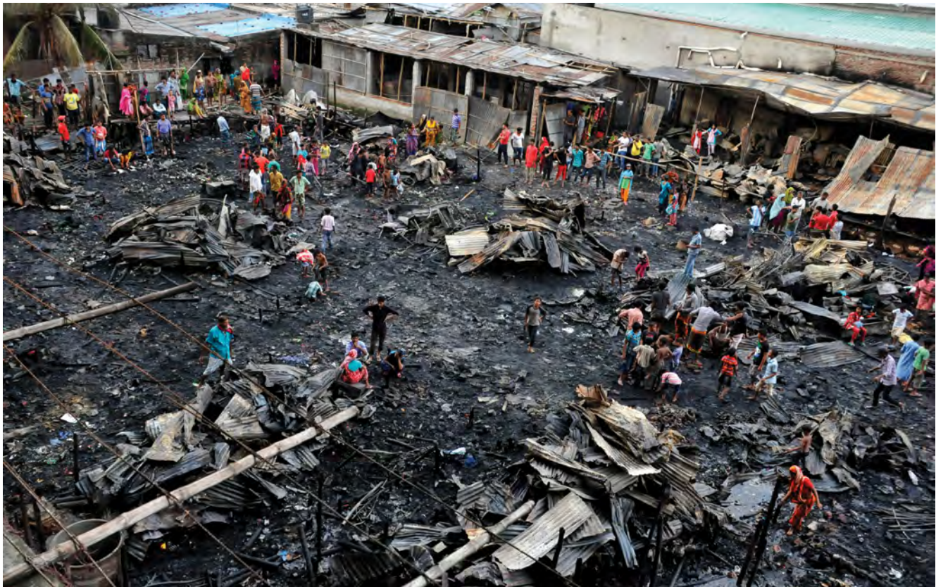
With structures packed tightly together in slums, fires can spread very quickly.
