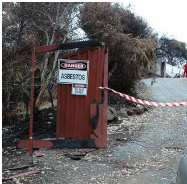
Access restrictions can arise when post-fire hazards are identified.
