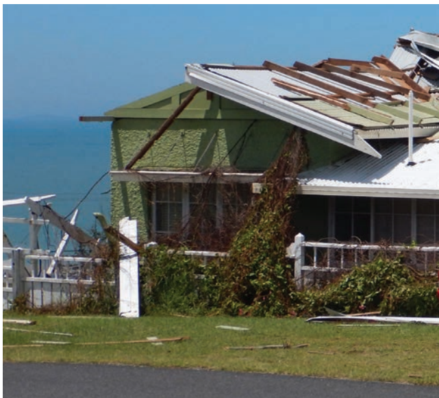
Severe roofing failure due to weak roof framing connections in properties happened during Cyclone Marcia in 2015 in Yeppoon, Queensland. Image: Cyclone Testing Station, James Cook University.
