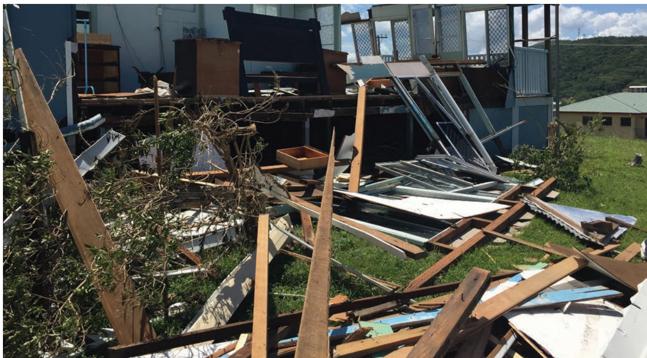
Cyclone Marcia caused significant damage to property in Yeppoon, Queensland due to its severe winds and the way properties were constructed. Image: Cyclone Testing Station, James Cook University.
