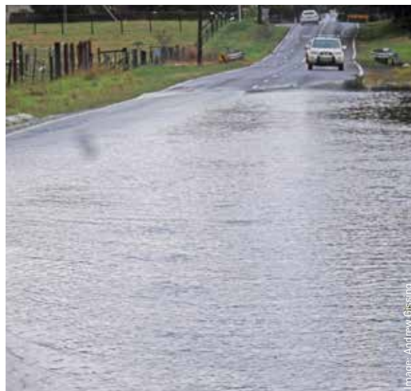
The research location included a local road closed by floodwaters. There were no depth markers or side railings along the section of flooded road.
