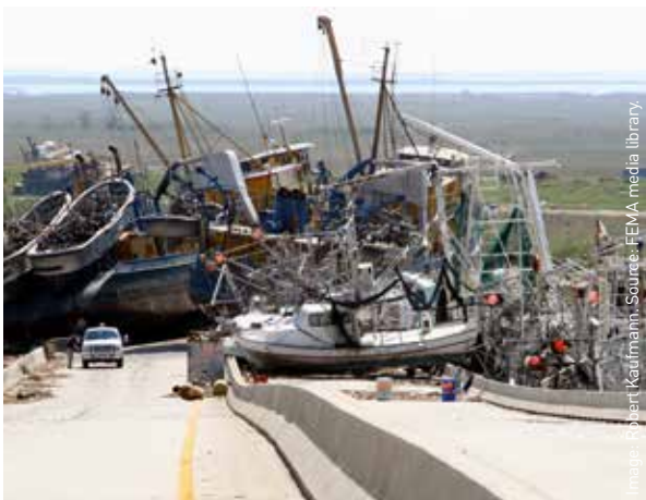
This bridge in Empire, Louisiana, was closed for almost 60 days after Hurricane Katrina went through the area in 2005.
