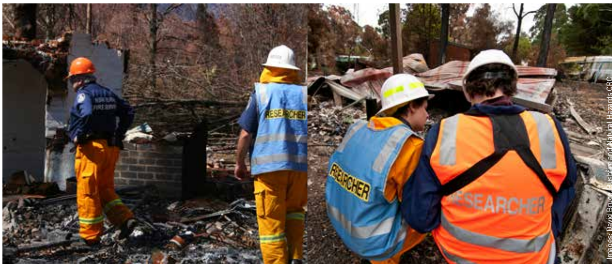
Researchers inspect property damage at Marysville and Kinglake after the 2009 Black Saturday fires in Victoria.
