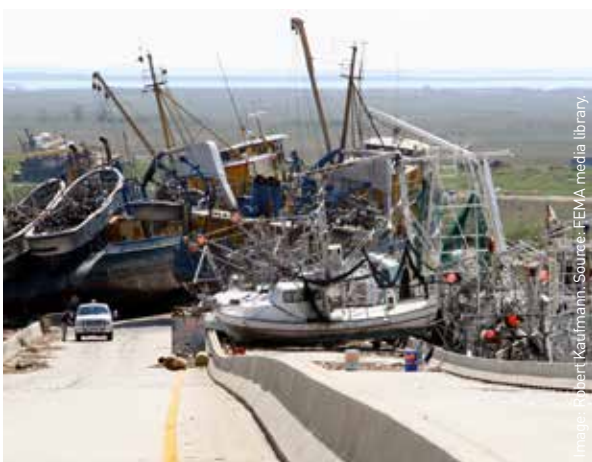
This bridge in Empire, Louisiana, was closed for almost 60 days after Hurricane Katrina went through the area in 2005.
