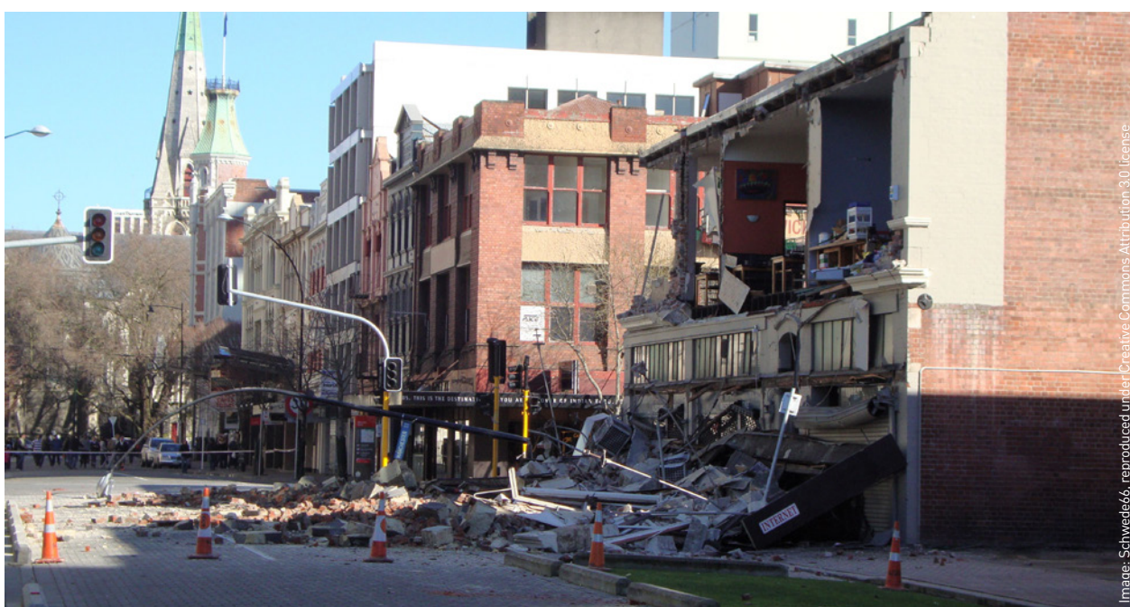
Earthquake damage on Worcester Street, Christchurch after the 2010 quake.
