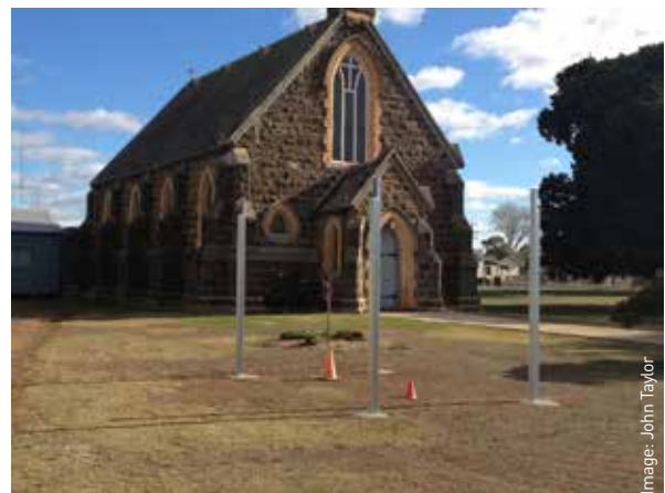
A new gazebo under construction.
