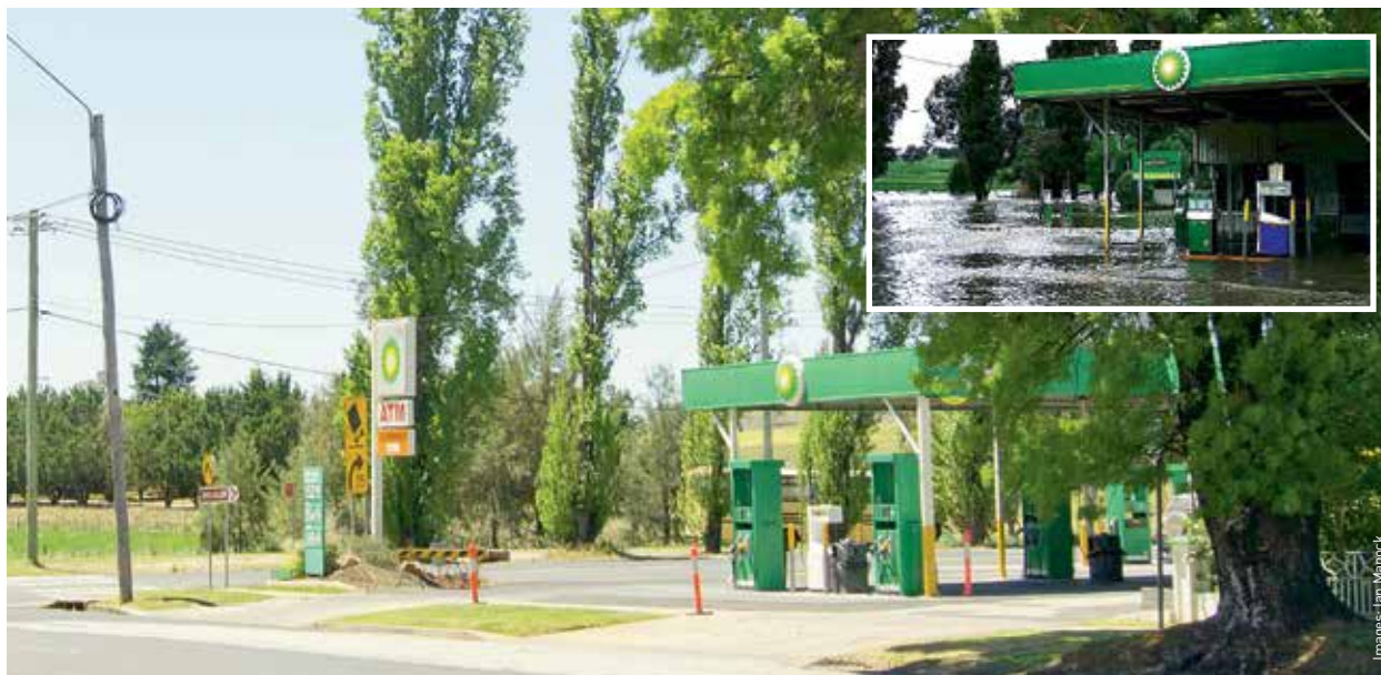
At the intersection of Gidley Street and Mitchell Highway floodwaters lapped the bottom of the petrol pumps at the BP Service Station.
