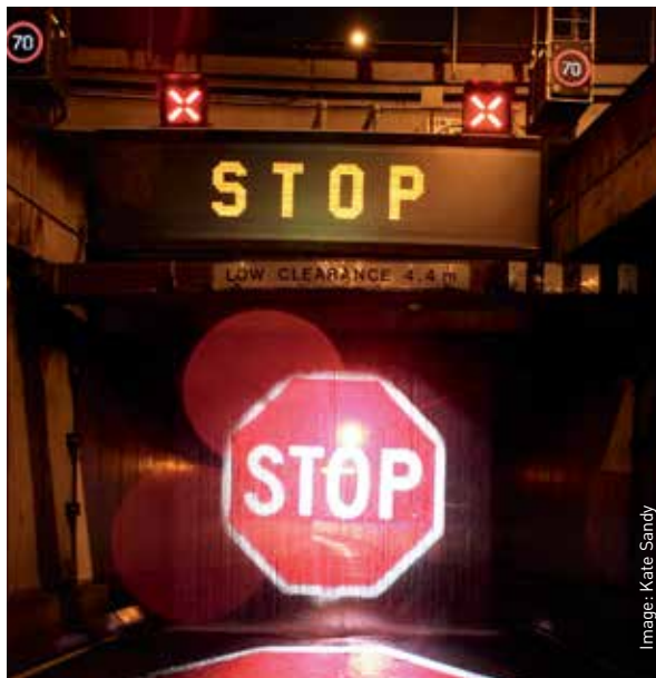
Stop sign at entrance to the Sydney Harbour Tunnel southbound carriageway. It was developed to stop motorists entering the tunnel after other warning signs had failed to achieve this. It consists of a cascading wall of water on which a stop sign is projected.
