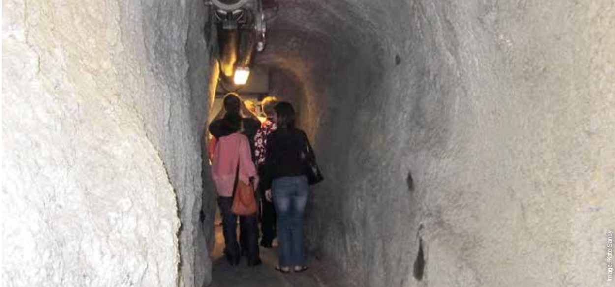
Exit cross tunnel, part of the evacuation route.
