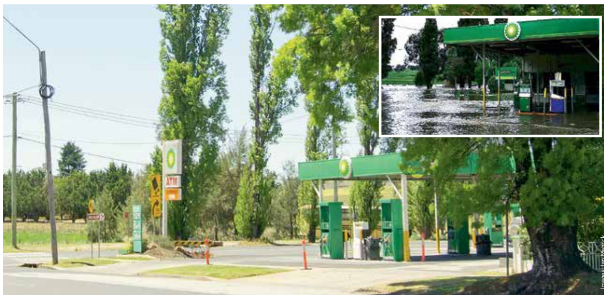
At the intersection of Gidley Street and Mitchell Highway floodwaters lapped the bottom of the petrol pumps at the BP Service Station.
