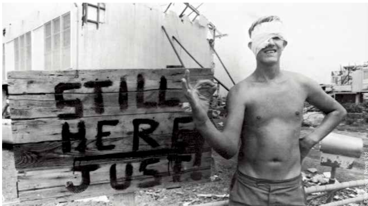
December 1974: Darwin, NT. An injured survivor of Cyclone Tracy stands in front of the wreckage of a building in Darwin.
