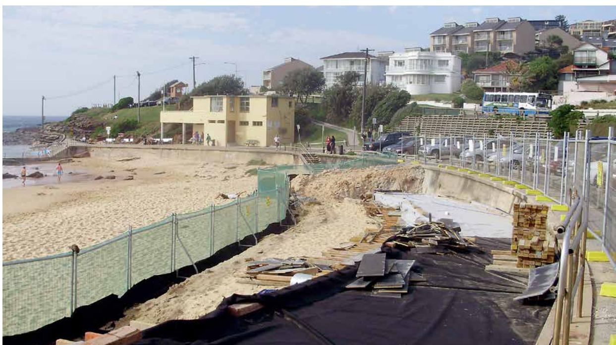
Reconstruction work on Collaroy Beach, Sydney, Australia.
