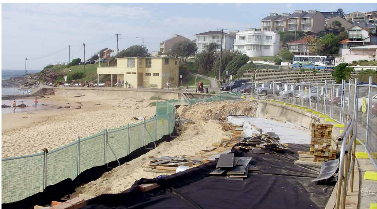
Reconstruction work on Collaroy Beach, Sydney, Australia.
