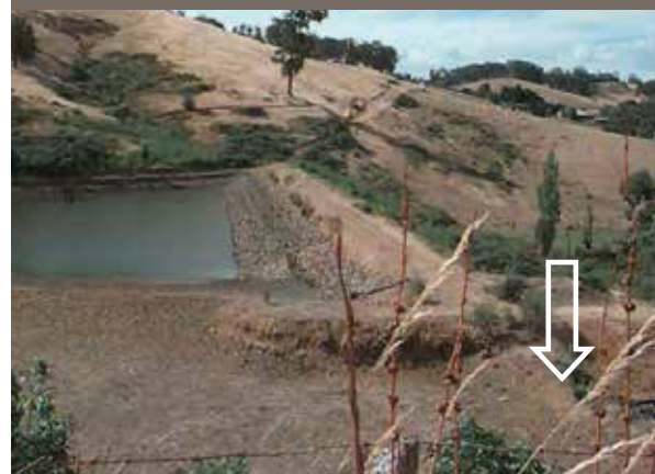
FIGURE 3. Dam No. 4 in 1995 showing the spillway blocked by a mound of dirt. There is also dense vegetation allowed to grow on the downstream face of the embankment.
