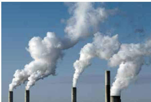
Hazardous airbourne pollutants.
