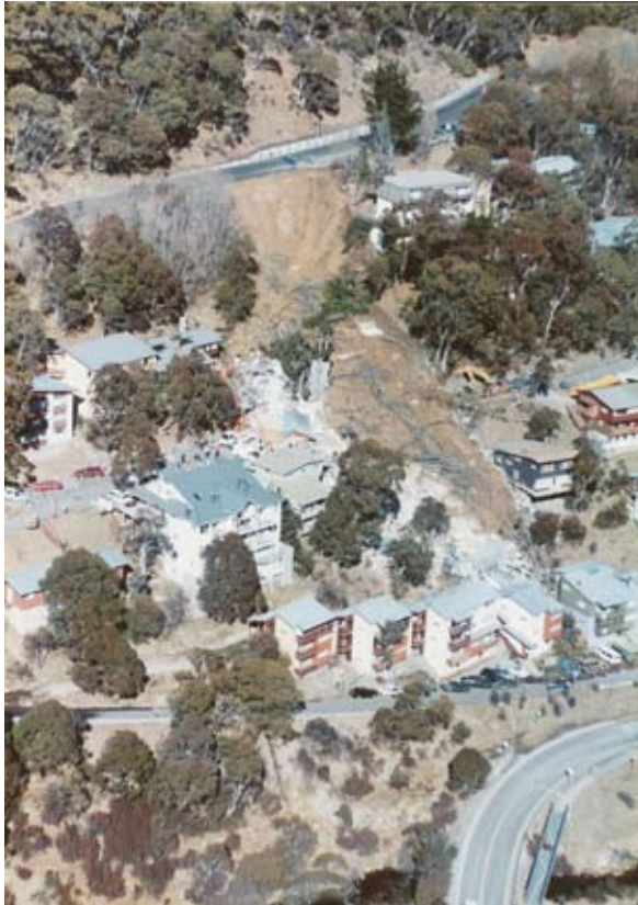
This landslide of 30 July 1997 at Thredbo claimed 18 lives as a consequence of the destruction of two ski lodges by a failure of the road embankment fill of the Alpine Way.
