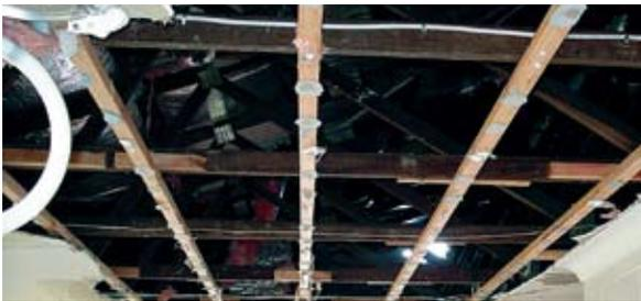
Figure 8: Ceiling damaged by water ingress from debris impact to gable
