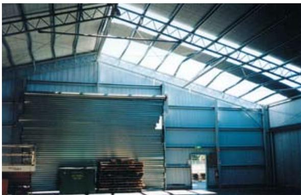
Figure 9: Structural failure of shed from failure of roller door on windward wall
