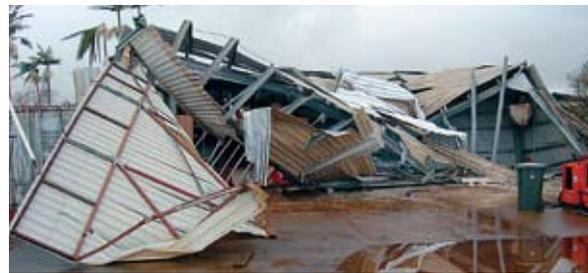
Figure 7: Failure of cold formed steel frame shed
