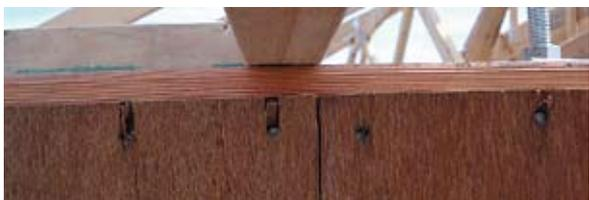
Figure 10: Gun nails over driven in bracing panel.
