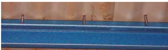
Figure 9: Roofing screws missed top hat batten.
