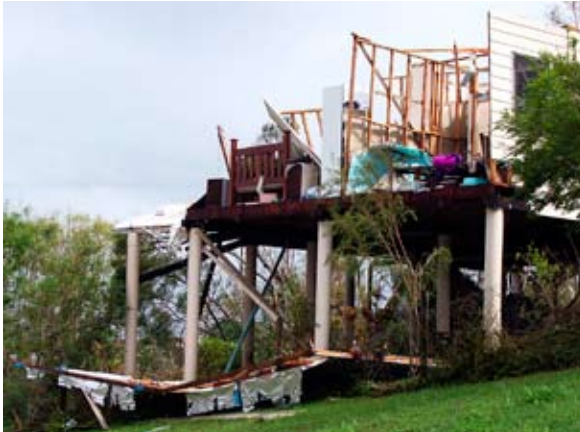
Figure 6: Elevated house on side of hill
