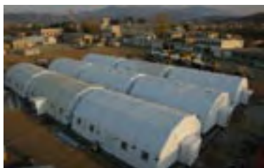
The MSF Inflatable tent hospital in Mansehra, North West Frontier Province (Pakistan) for the October 2005 earthquake. © Remi Vallet / MSF.
