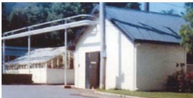
Boiler room and hot house
