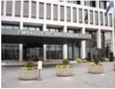
Embassy of Australia in Washington DC
