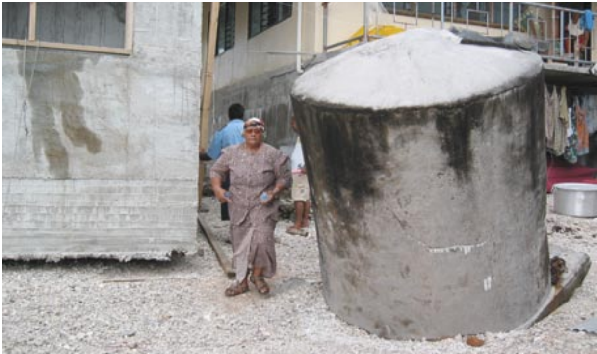
Beach erosion exposed house foundations and moved water tanks on Nukunonu.
