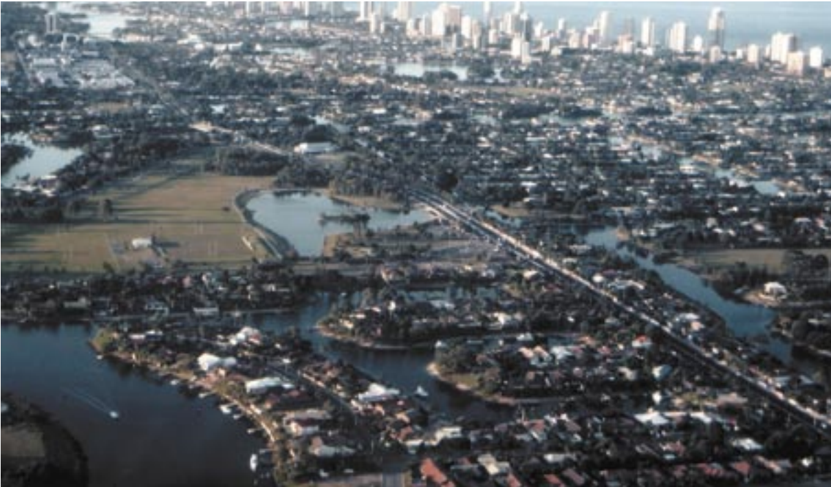
Looking northeast across the floodplain in 2002 – development today (Photo courtesy of O. Harvey).
