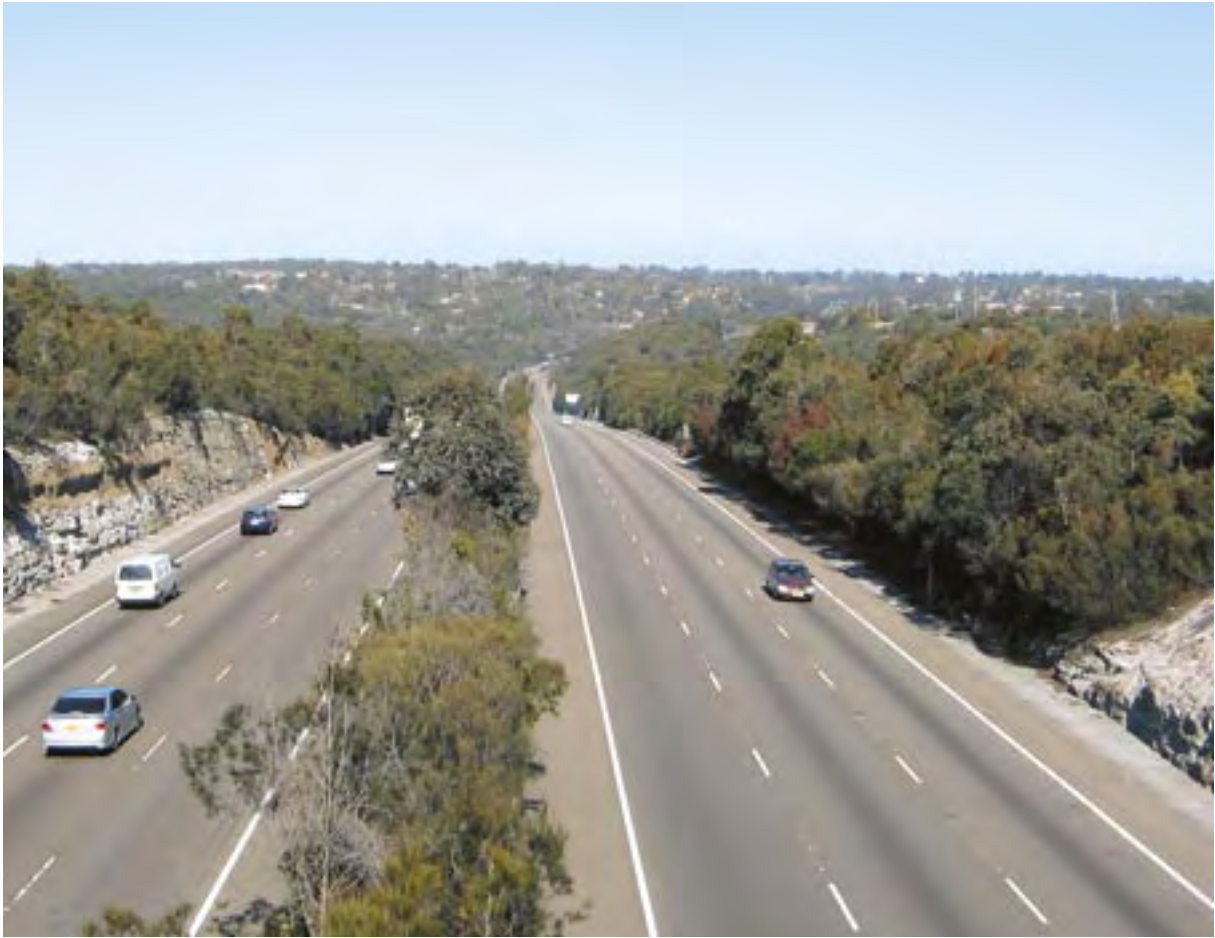
The Sydney – Newcastle Freeway (F3) is often closed due to severe smoke and bushland fires surrounding the road during peak seasons. As this is the only main roadway linking Sydney to Newcastle, extensive delays occur.
