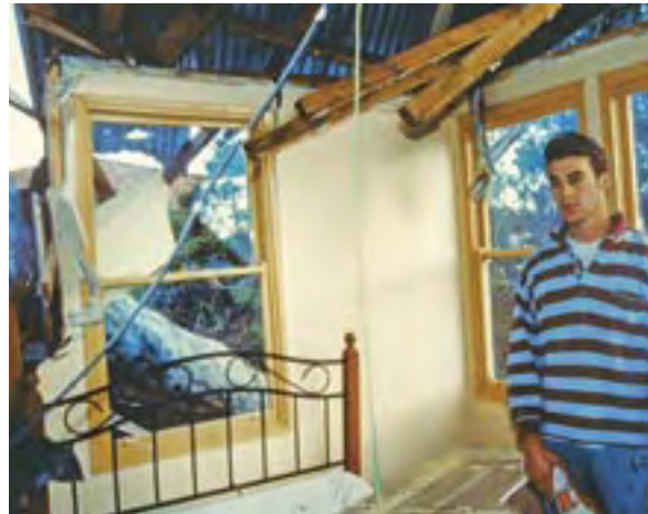
The risk of damage to a house and injury to its inhabitants can be minimised by securing the roof and internal fixtures such as high bookcases and mirrors
