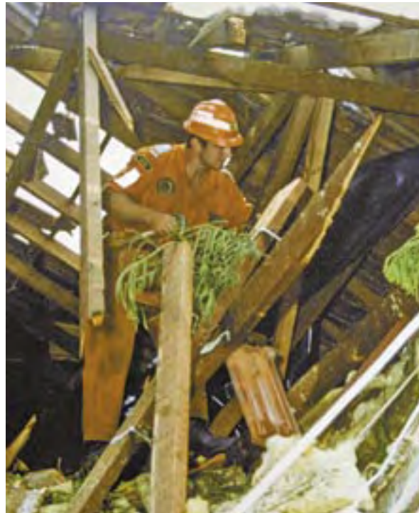
Damage to buildings and infrastructures are only a part of disaster loss assessment
