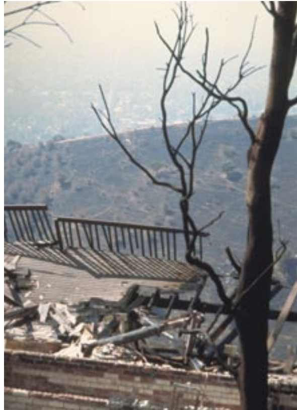
Fire retardation qualities are not well incorporated into building and planning practices
