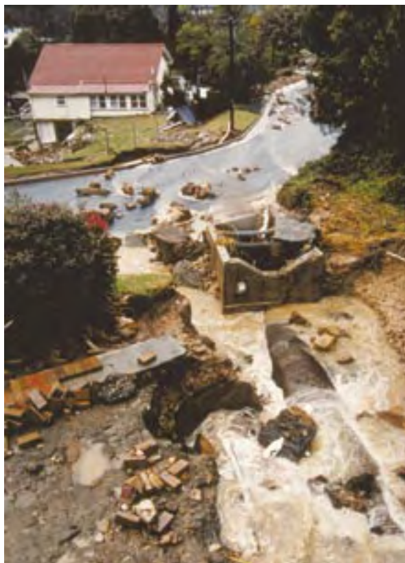
Landslides affect infrastructure and recovery processes for emergency workers and survivors
