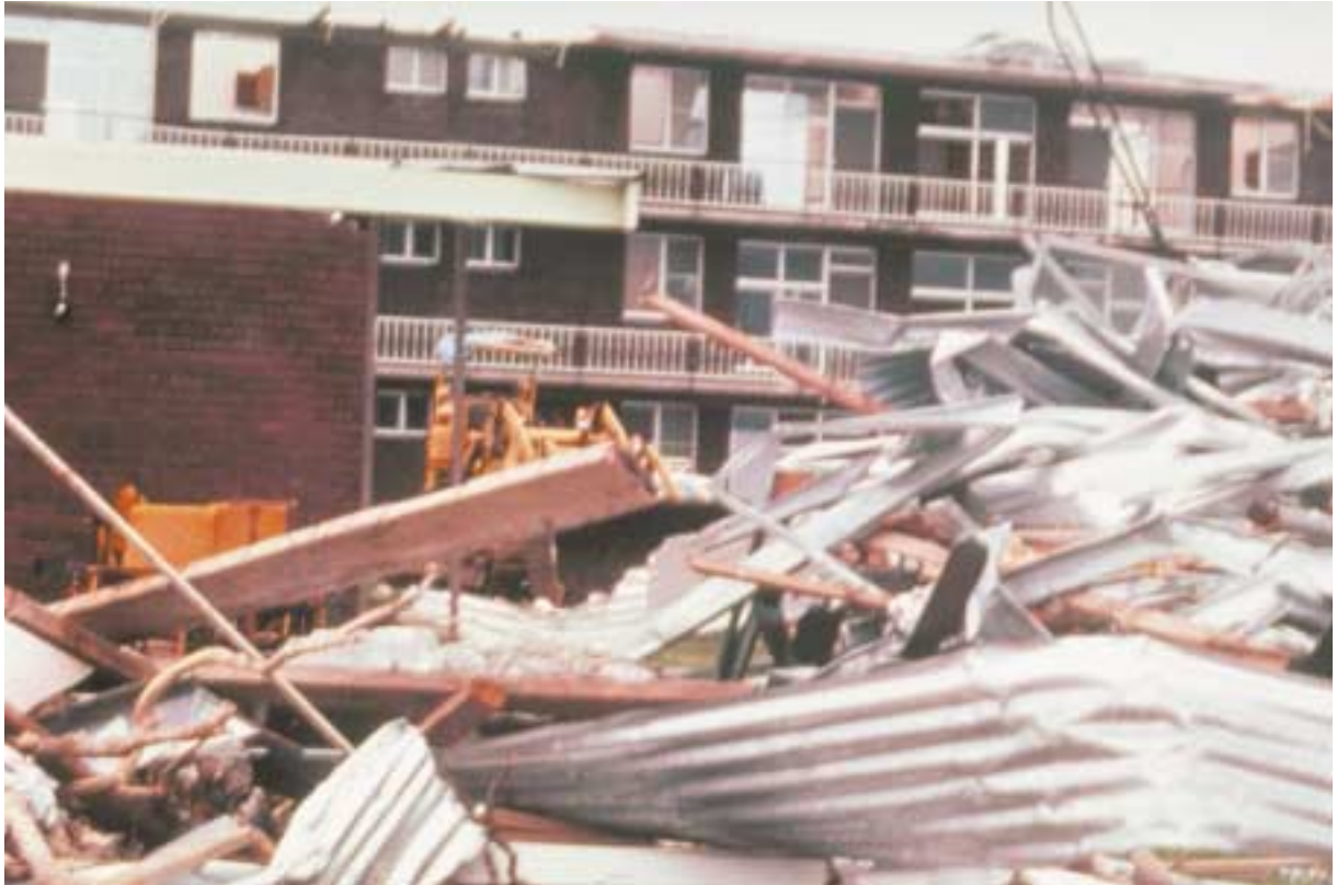
Structural inadequacy is exposed by failure of so many buildings. Compare for instance the building in the rear to the building in the foreground
