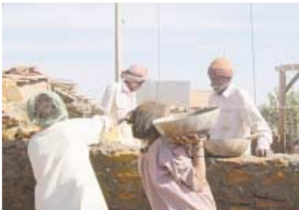
Figure 7: Family builds its own house
