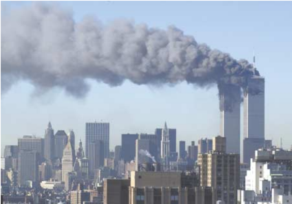
The World Trade Centre burns after the terrorist attacks in September 2001.
