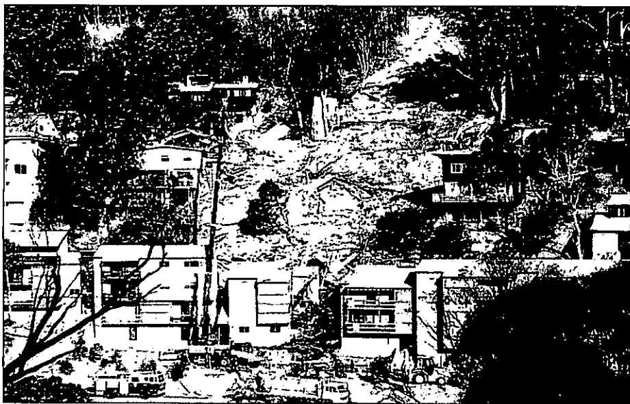
Figure 1: Top – Thredbo Village disaster domain before the 30 July 1997 landslide, looking towards Bimbadeen and Carinya Lodges (arrowed). Below – after the landslide.
