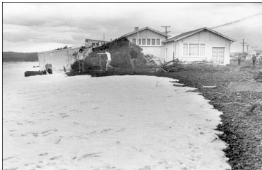
Figure 3: Houses in danger (between Haumoana and Te Awanga) 1974.
