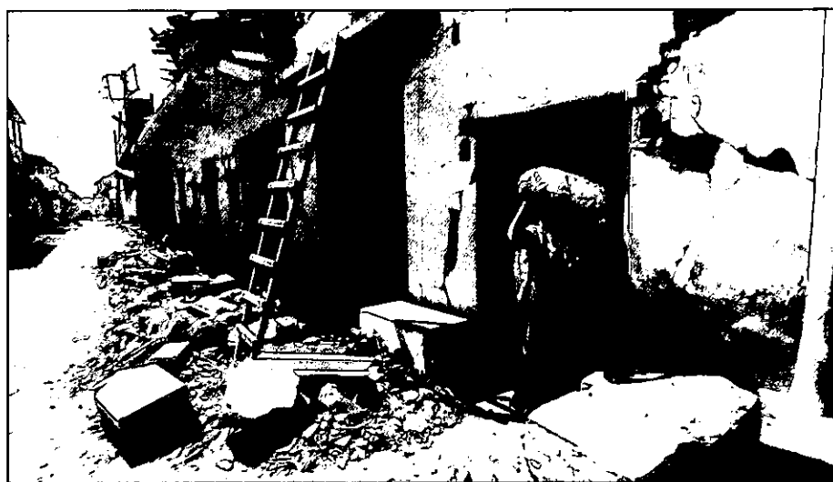
top: In El Salvador, many homes were lost beneath a wall of debris from a collapsing slope above. above: In Gujarat, the earthquake didn't kill, but the buildings did. (images courtesy International Federation of Red Cross and Red Crescent Societies)
