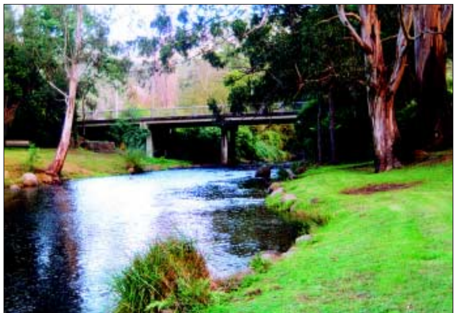
Figure 3: The Blackwood Avenue landslip lies on the north bank of the Yarra River at Warburton. The toe of the landslide is at the edge of the river. In the unlikely event of a total blockage of the river, infrastructure such as the bridge spanning the Yarra River could be affected.
