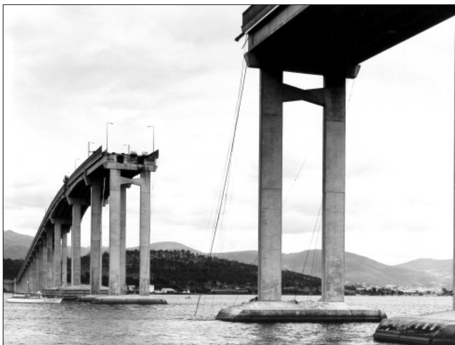
Figure 3 – Tasman Bridge, 6 January 1975
