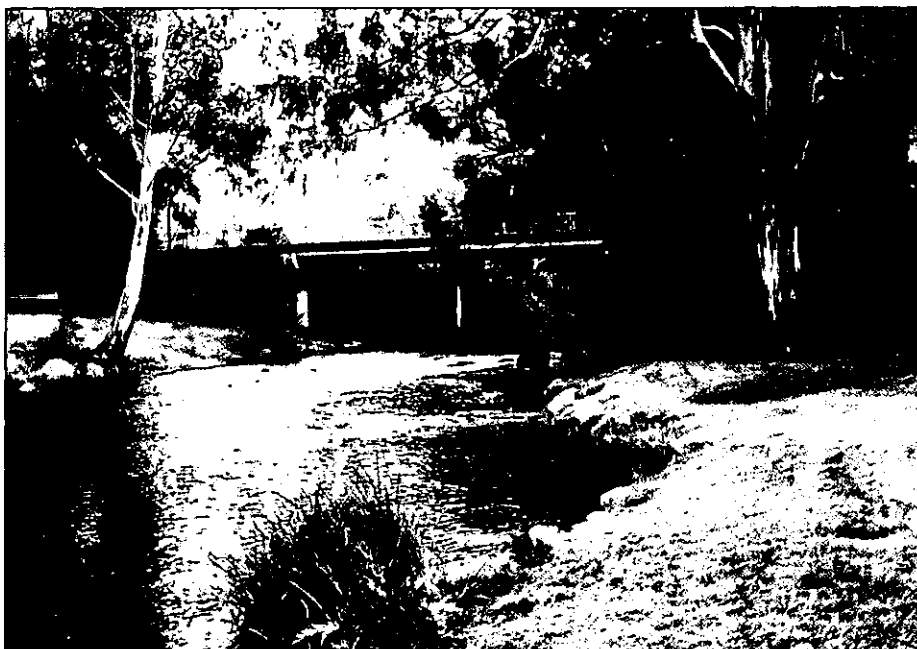
Figure 3: The Blackwood Avenue landslide lies on the north bank of the Yarra River at Warburton. The toe of the landslide is at the edge of the river. In the unlikely event of a total blockage of the river, infrastructure such as the bridge spanning the Yarra River could be affected.
