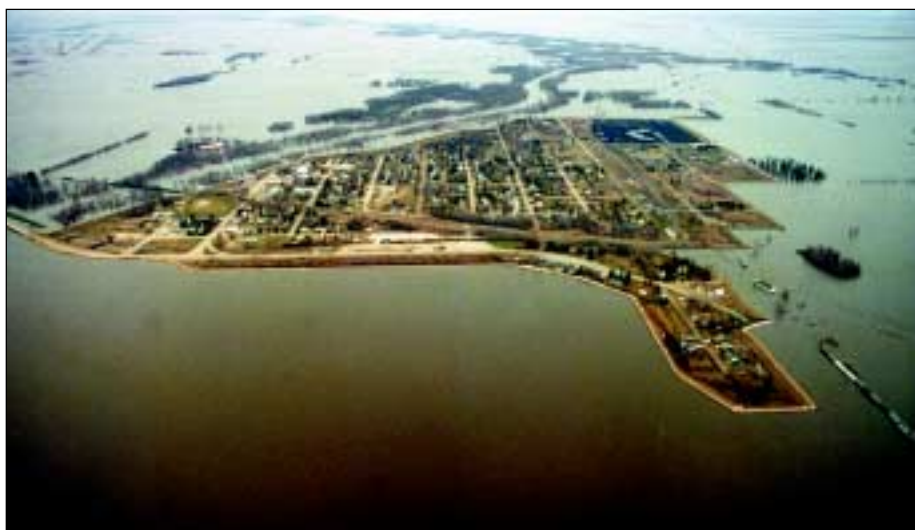
Figure 4: Aerial view of Emerson, Manitoba and Noyes, Minnesota, two communities within the transborder ring-dike. The American area is the lower portion extending downward. Photo courtesy of Manitoba Conservation, Water Resources Branch.
