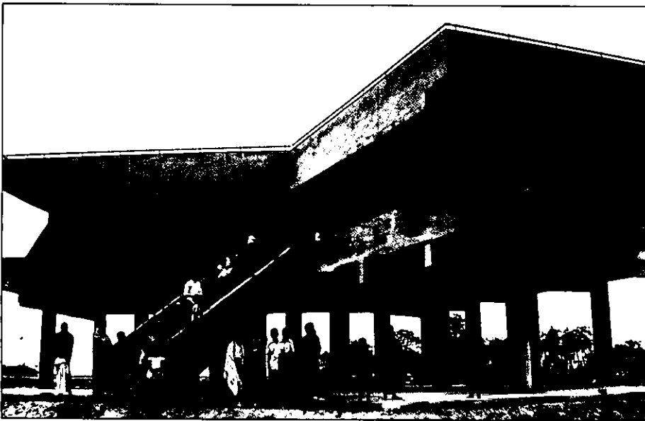
Above: a cyclone shelter in Bangladesh that has protected the lives of hundreds of vulnerable rural people living along the coastal Bay of Bengal.
