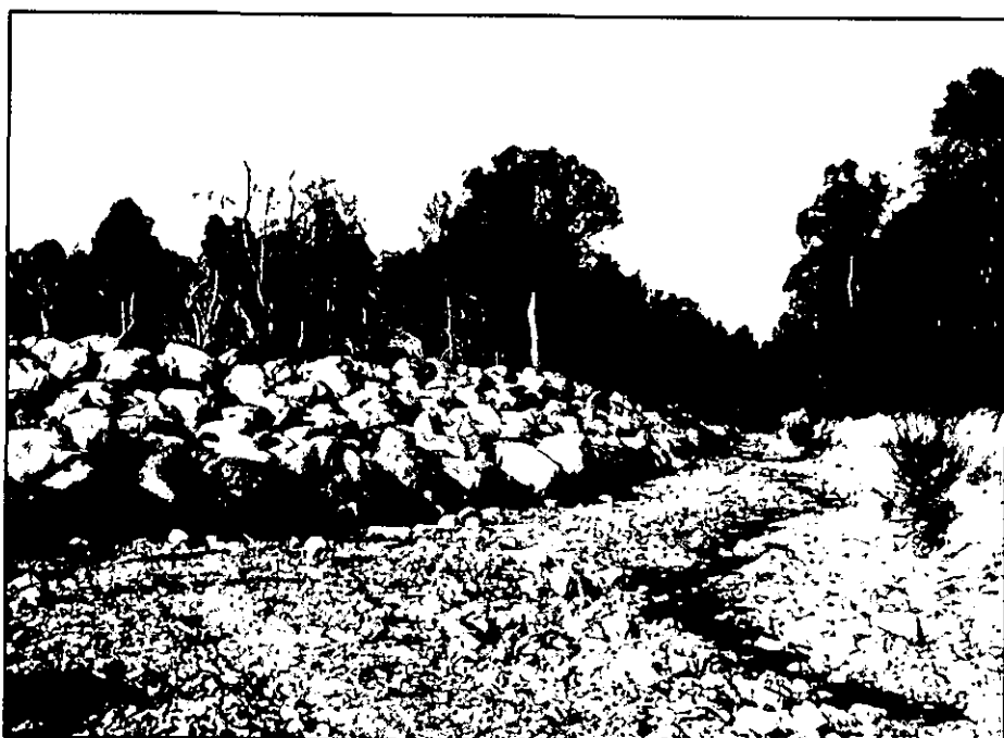
Figure 2(a): Kowhai Stream in 1985 showing the recently completed protective works.
