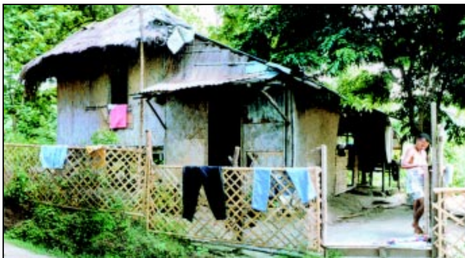
Figure 4: A typical housing unit constructed in bamboo and grass or nipa, an accommodation provided by the government to Aetas in the Upland Resettlement Site as a permanent post-disaster shelter.
