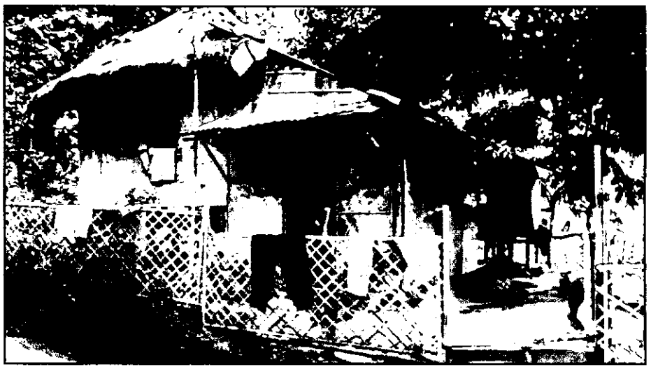
Figure 4: A typical housing unit constructed in bamboo and grass or nipa, an accommodation provided by the government to Aetas in the Upland Resettlement Site as a permanent post-disaster shelter.
