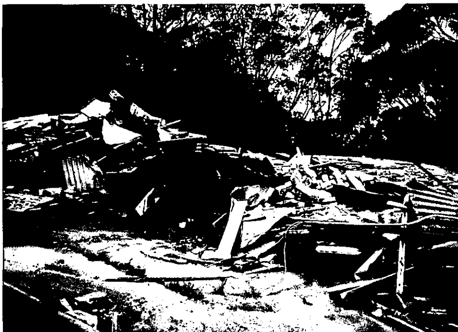
This old mine building on Mt Keira was destroyed by a debris flow during the Wollongong floods in August 1998.
