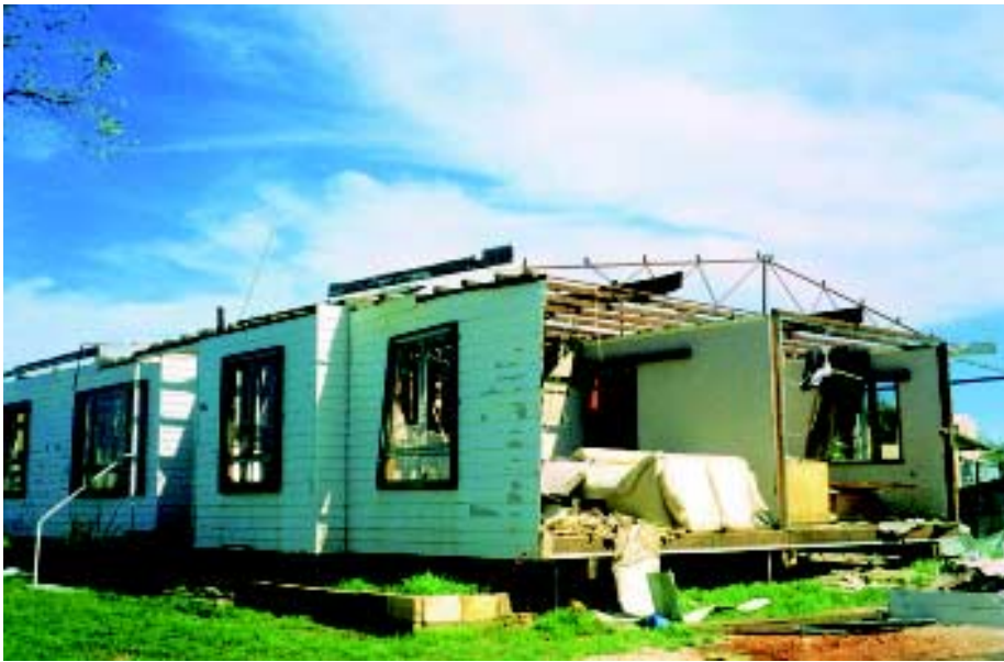
Photo 2: Transportable houses put in the poorest performance of any housing group.
