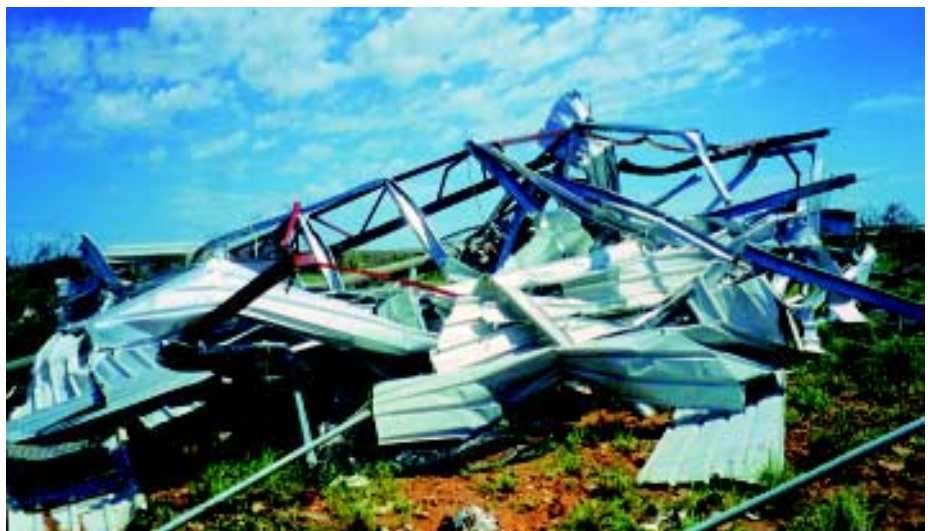
Photo 6: This entire building became flying debris, coming to rest wrapped around a light pole.
