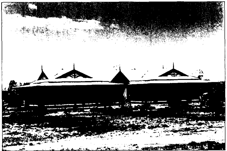
Photo 1: The majority of newer houses successfully resisted the wind forces.
