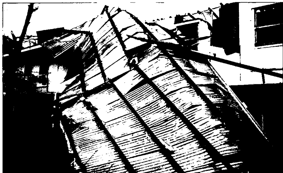
Photo 4: On this block of flats, the leeward roof slope peeled off in one piece, initiated by failure near the ridge.
