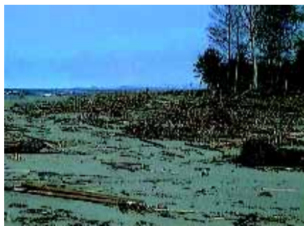
Coastal zone after tsunami impact
