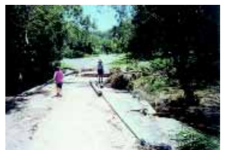
Photo 2: Barton St. bridge, breached by flood waters, Nelly Bay.
